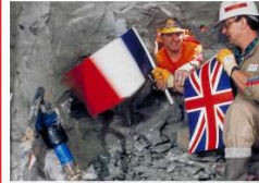
Channel Tunnel (Chunnel) , England-France
